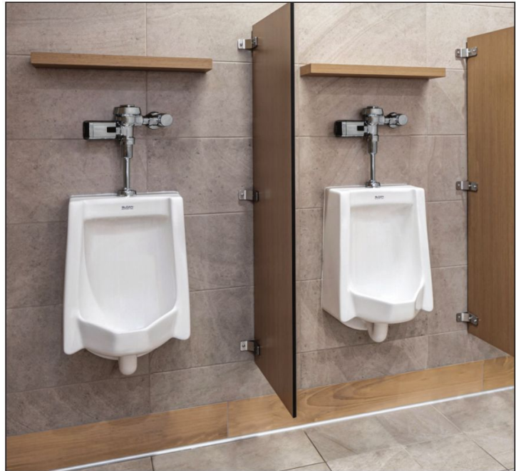
Sensor flushometers, equipped with reclaimed water features, are designed to withstand the harsh conditions presented by reclaimed water while conserving water at the same time.
